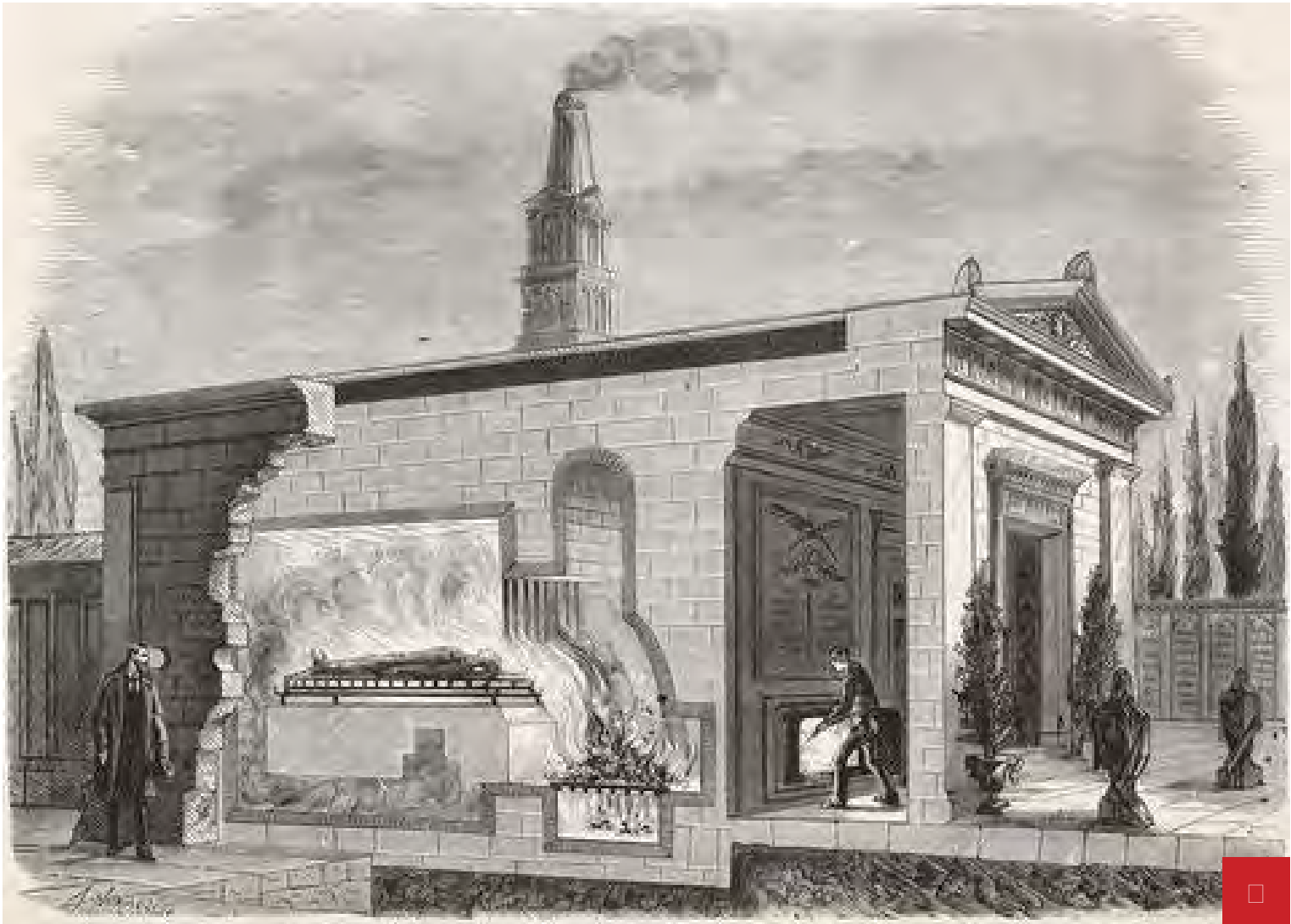
Garinis cremation furnace, Milan, Italy, illustration from Lllustration, Journal Universel, No 1965, Volume LXXVI, October 23, 1880
